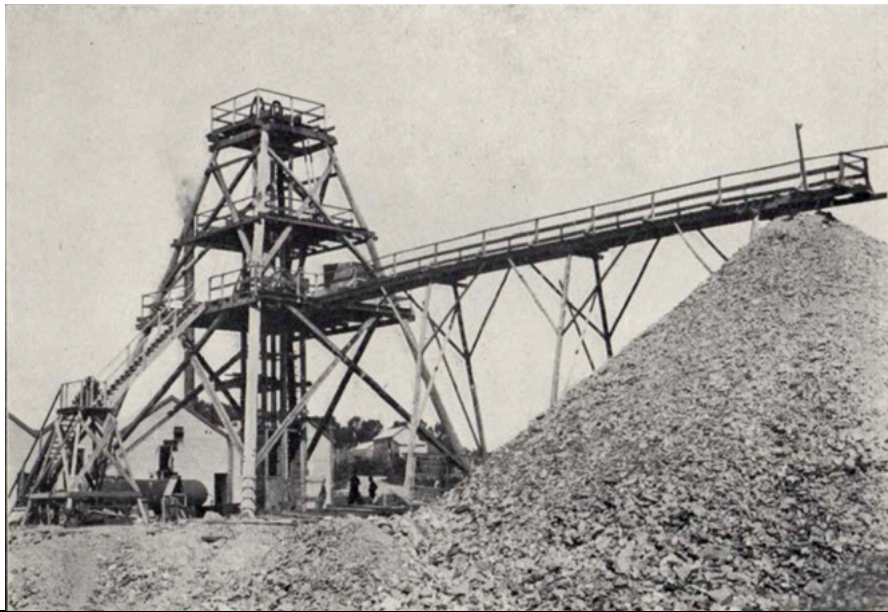
Figure 38: A typical headframe (or poppet legs), Daylesford
